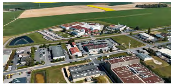
AXON' HEADQUARTERS /France
